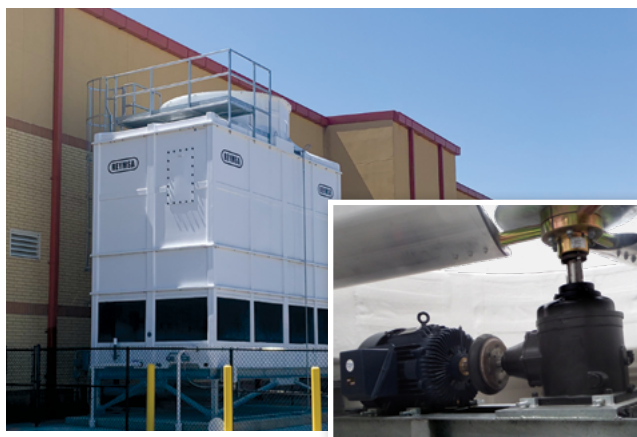
Single fan model Standard: Gear Drive System
