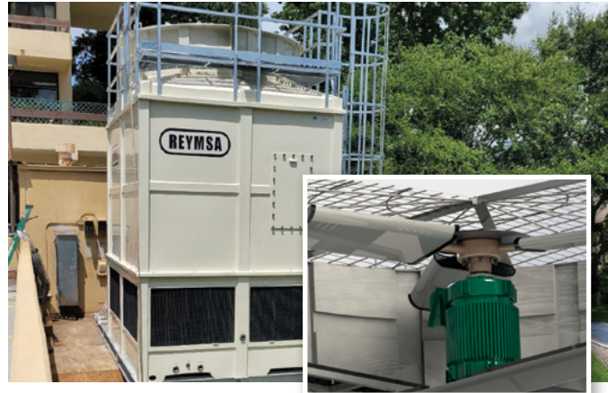
Single fan model Optional: Direct Drive System
