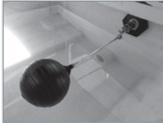
Figure AP-1: Float valve installed in a cooling tower
