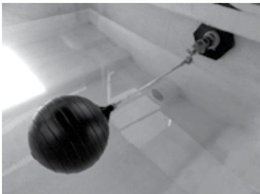
Float valve installed in a Cooling Tower
