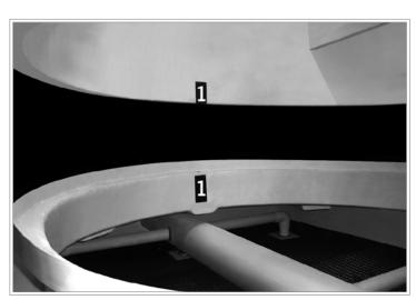
Figure A-37: Fan adaptor alignment
