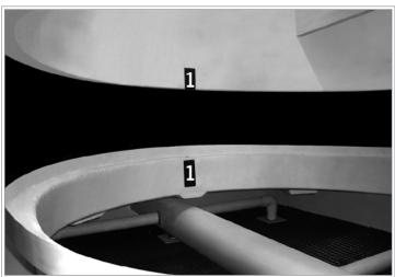
Figure A-27: Fan duct alignment for a four fan tower
