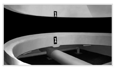
Figure A-17: Fan duct alignment for a double fan tower
