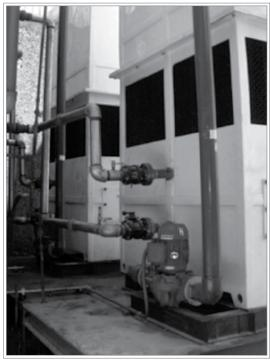
Figure A-63: Example of a base support (provided by others)
