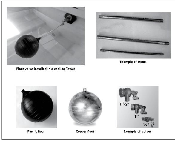
Figure AP-1: Float valve parts
